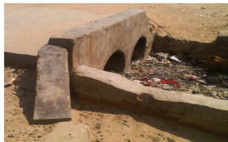
**Plate 2:** Blockage of Drainage Channel in Bosso
