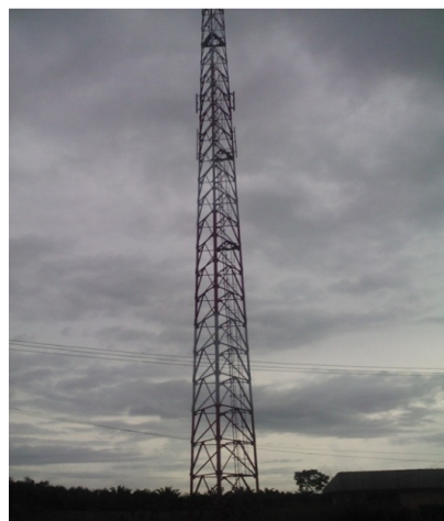
Fig.1 (a) Square-base self-supporting antenna tower (courtesy:Nigerian Telecommunication Ltd).
