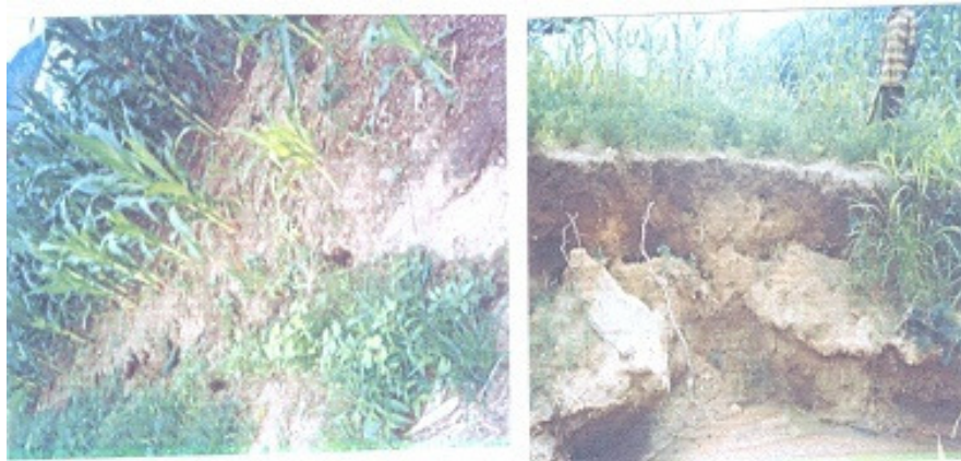
Plate 3: Gully erosion at farm level
