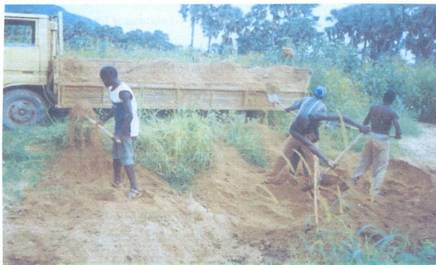
Plate 1. Sand mining accelerates Gully erosion in the area
